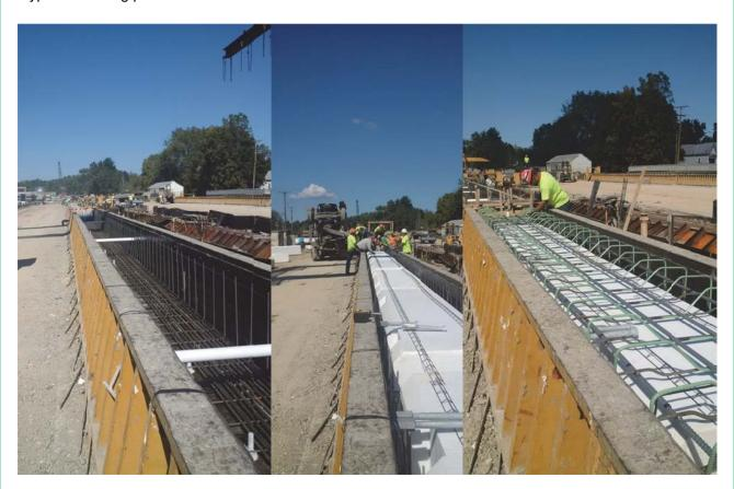
The pictures above provide a review of one example of Plasti-Fab EPS being used to form a void within a concrete bridge beam and illustrate the following points:
